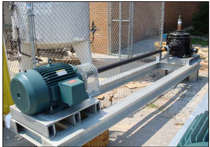
Fig. 2 Typical Fan Drive Arrangement
